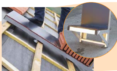
Rolls to slide trolley along lathing
